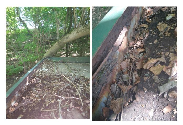
**Item 1** – The roof has corroded and is no longer watertight. The tree is growing around the structure exerting force onto the building.
