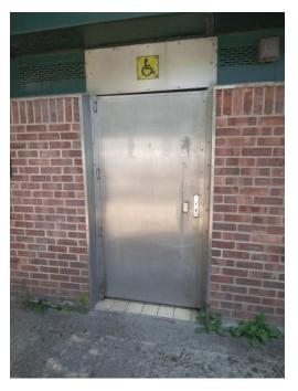
**Item 3** – The brickwork is also distorting at the top and the door no longer closes in this corner. Also, you can see the gaps at the tops of the door, how uneven the building is. Aspirational for our people, our place and ourselves
