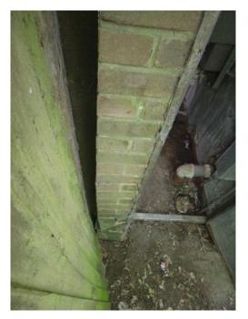
**Item 2** – At the rear of the building, there is a crack running down the middle. In the bottom right-hand corner, the brickwork is distorting at the bottom and top.
